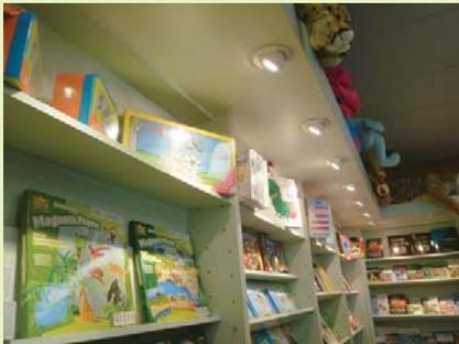
**Figure 1.** LED’s retrofit into halogen fittings in the Retail shop at Melbourne Zoo
